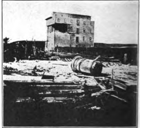
FIG. 137. — Damage caused by a Tornado at Rochester, Minn., August 21, 1883.
