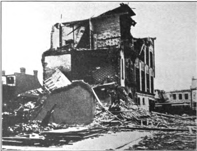
FIG. 138. — Wreckage of Anchor Hall, Jefferson and Park Avenues, St. Louis, May 27, 1896.
