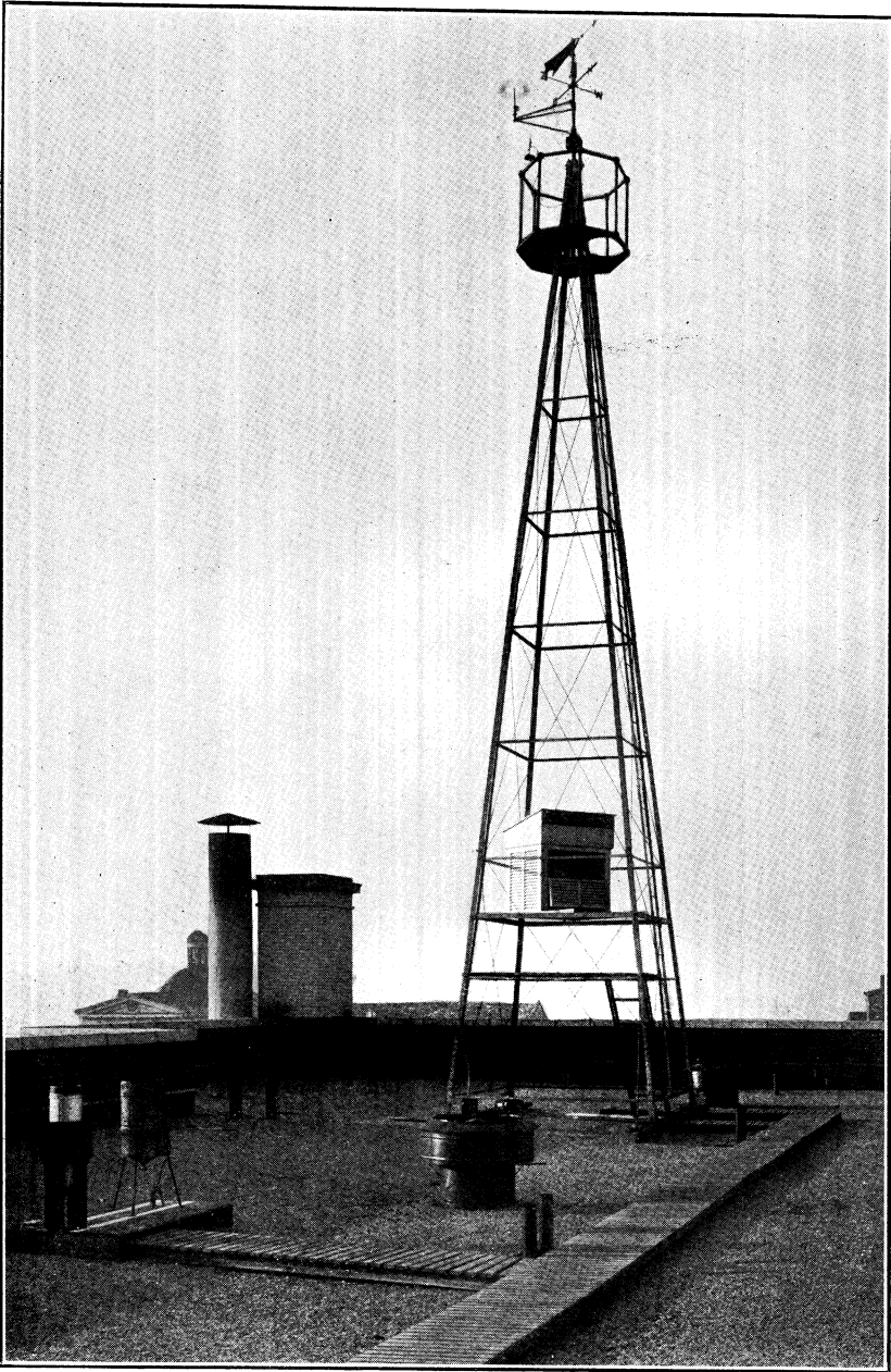
FORTY-FOOT STEEL WIND INSTRUMENT TOWER; TYPICAL INSTALLATION FOR HIGH OFFICE BUILDING. (LYNCHBURG, VA., JANUARY, 1914.)
