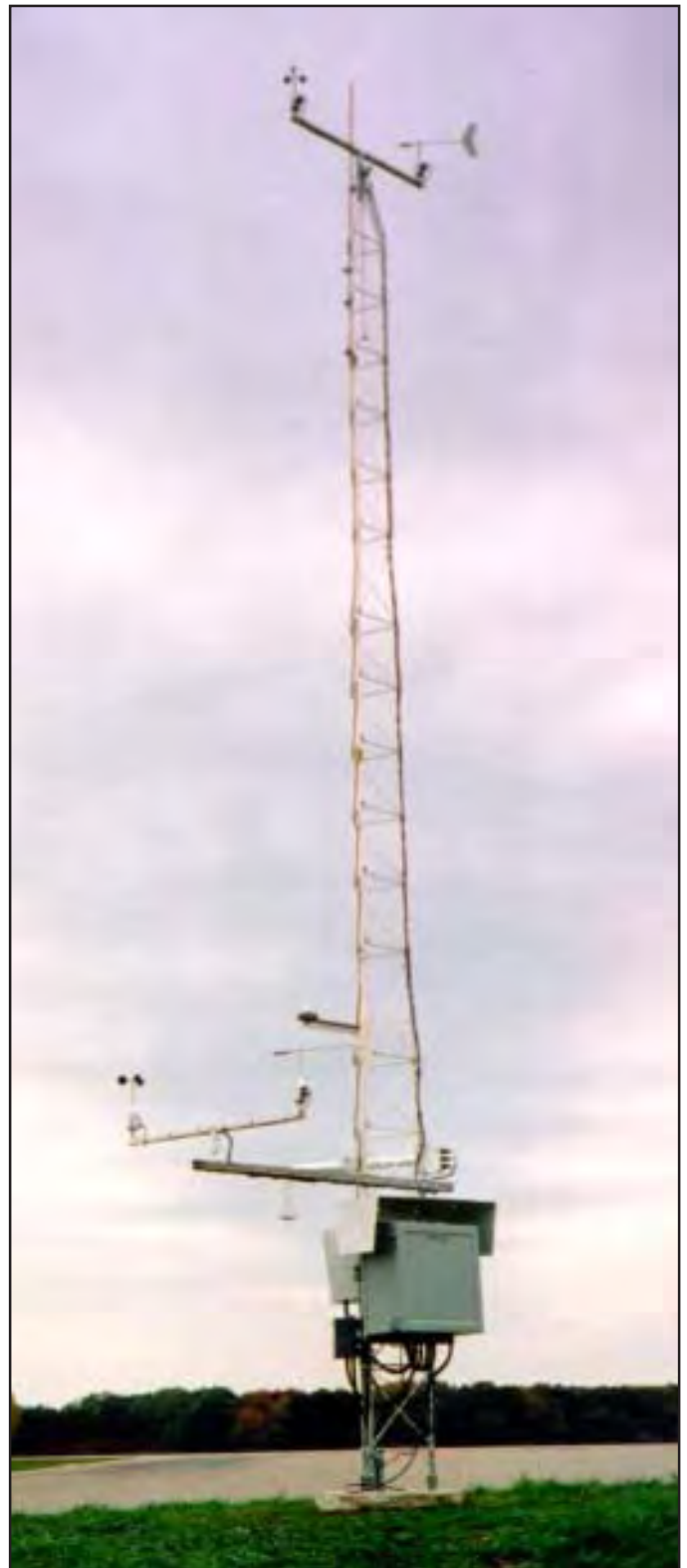
Tower-Mounted Meteorological Monitoring System
