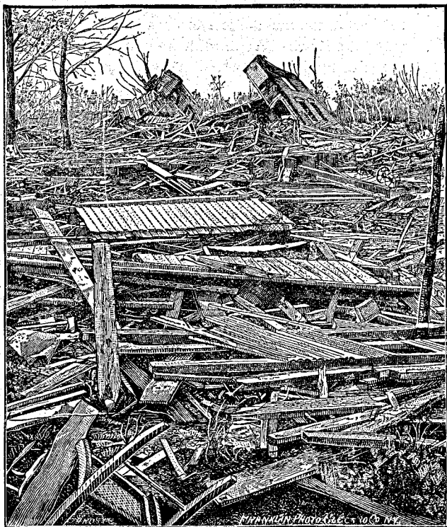
Tornado at Grinnell, Ia., June 17, 1882. General view looking in direction taken by the storm. From a Photograph. Dr. Grinnell's house in background. Shadow under the floor shows the place from which he took his wife and four children unharmed.
