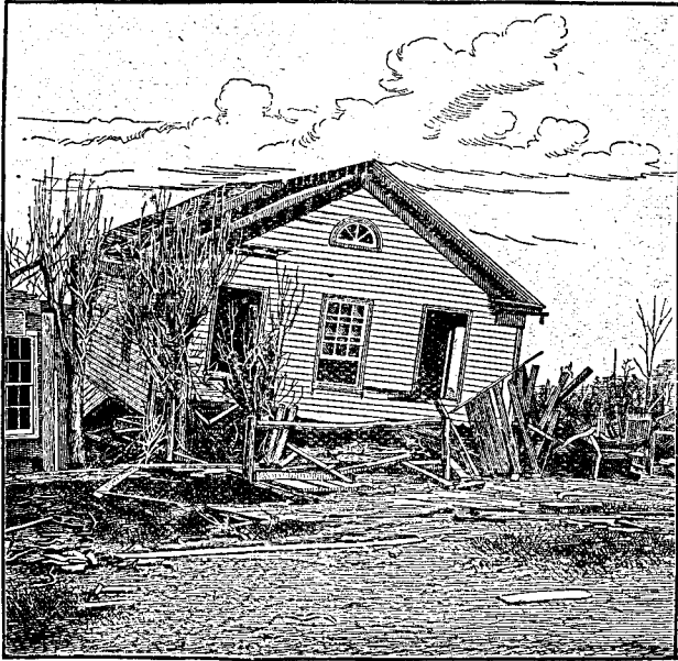
Tornado at Racine, Wis., May 18, 1883. House twisted from its foundation. From a Photograph.
