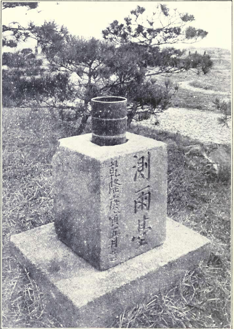
FIG. 80. THE OLDEST RAIN GAUGE This rain gauge was erected at Taiku in 1770.
