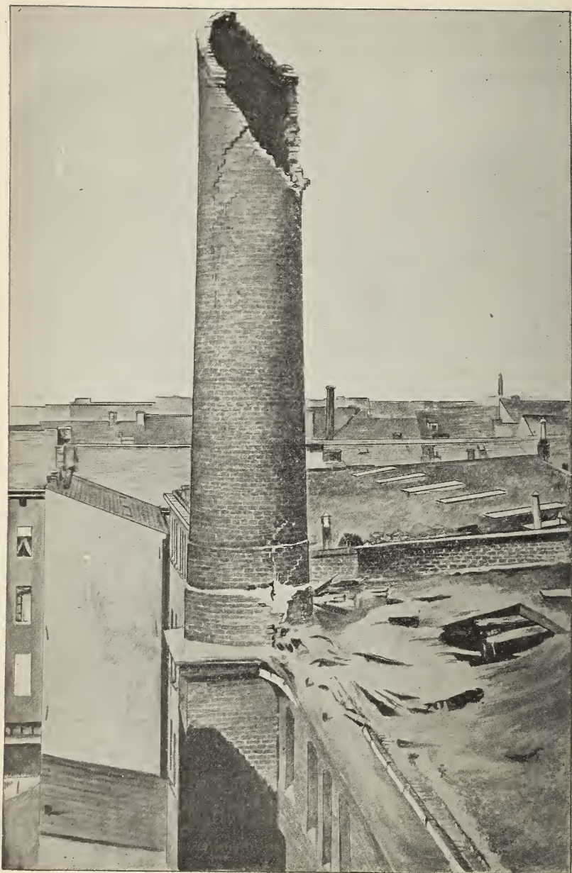
CHIMNEY, STRUCK JULY 29, 1890. From Elec. Zeits., Grebel.
